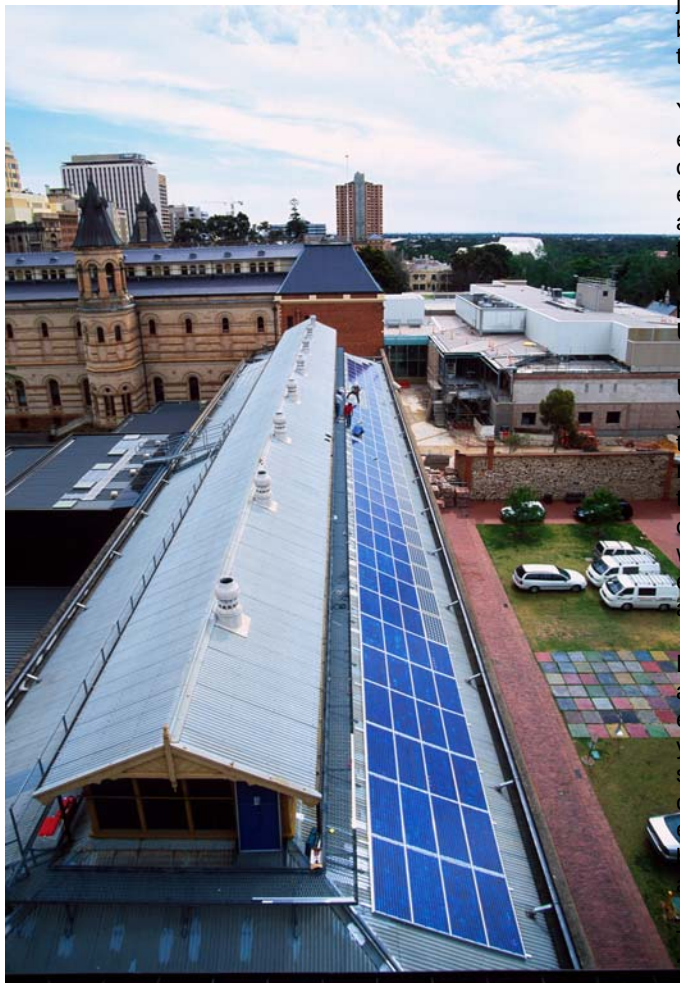
South Australia's solar powered museum. Image courtesy of SA Museum
